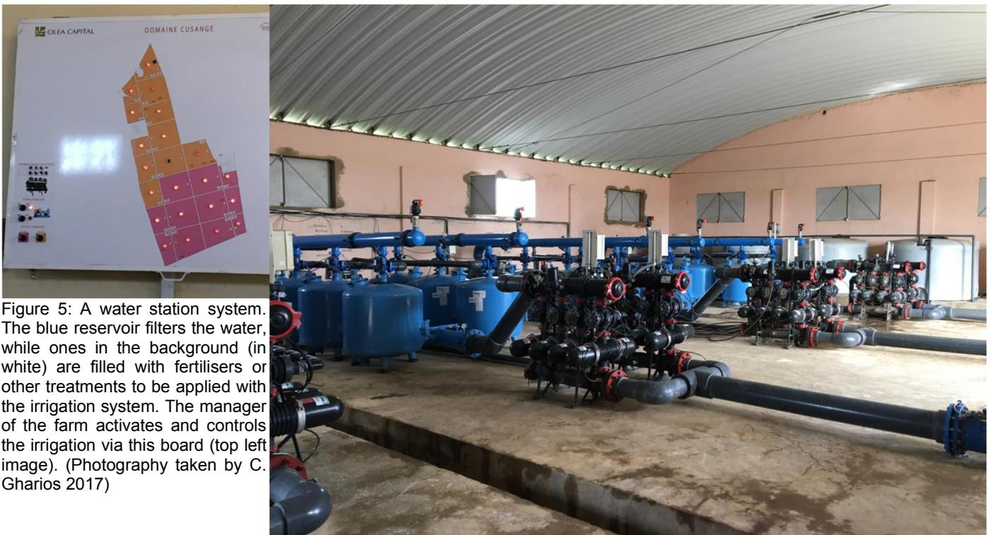
Figure 5: A water station system. The blue reservoir filters the water, while ones in the background (in white) are filled with fertilisers or other treatments to be applied with the irrigation system. The manager of the farm activates and controls the irrigation via this board (top left image). (Photography taken by C. Gharios 2017)
